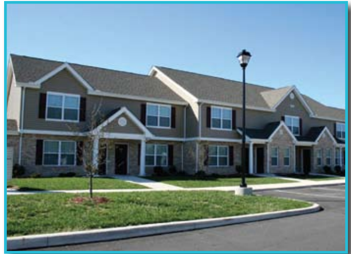
Old Landing II Apartments ~ Millsboro, DE ~ 30 Units
